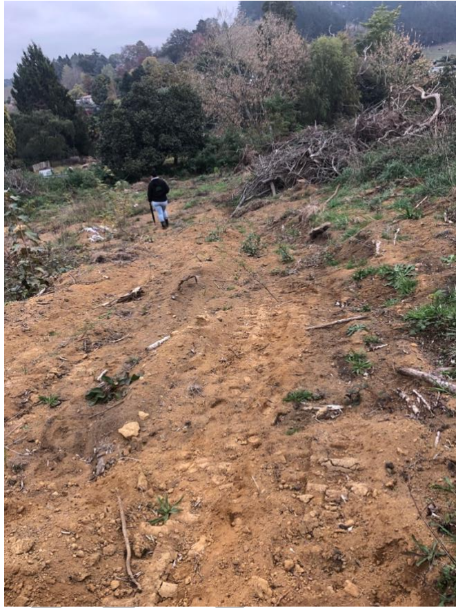
(Track above the excavated part of hill, Ngāwhare May 2022)
